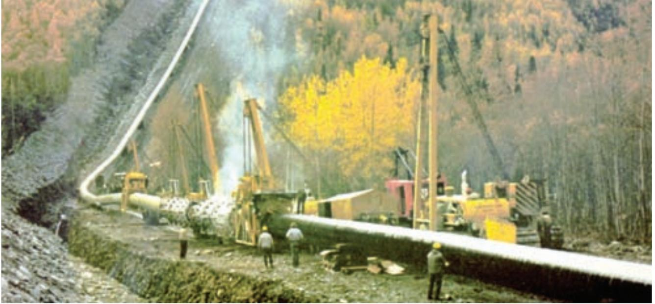
*Response to the 1970s' oil crisis—laying a below-grade section of the Alyeska pipeline (1.2 m OD, 605 km soil anchored, 60°C operating temperature) with Berejka's development of an EB-crosslinked, heat-shrinkable tape corrosion protection, Arcti clad II, in operation since 1975.*
