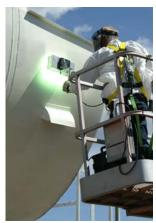
Figure 3. Field Application And Cure Of High Performance UV Coating Technology
