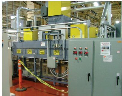
Thermal oven system.
