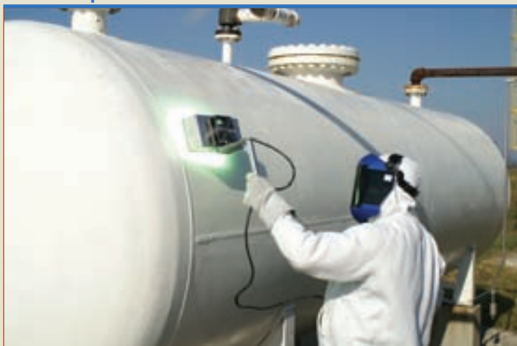
Field application and cure of UV technology at cold temperatures
