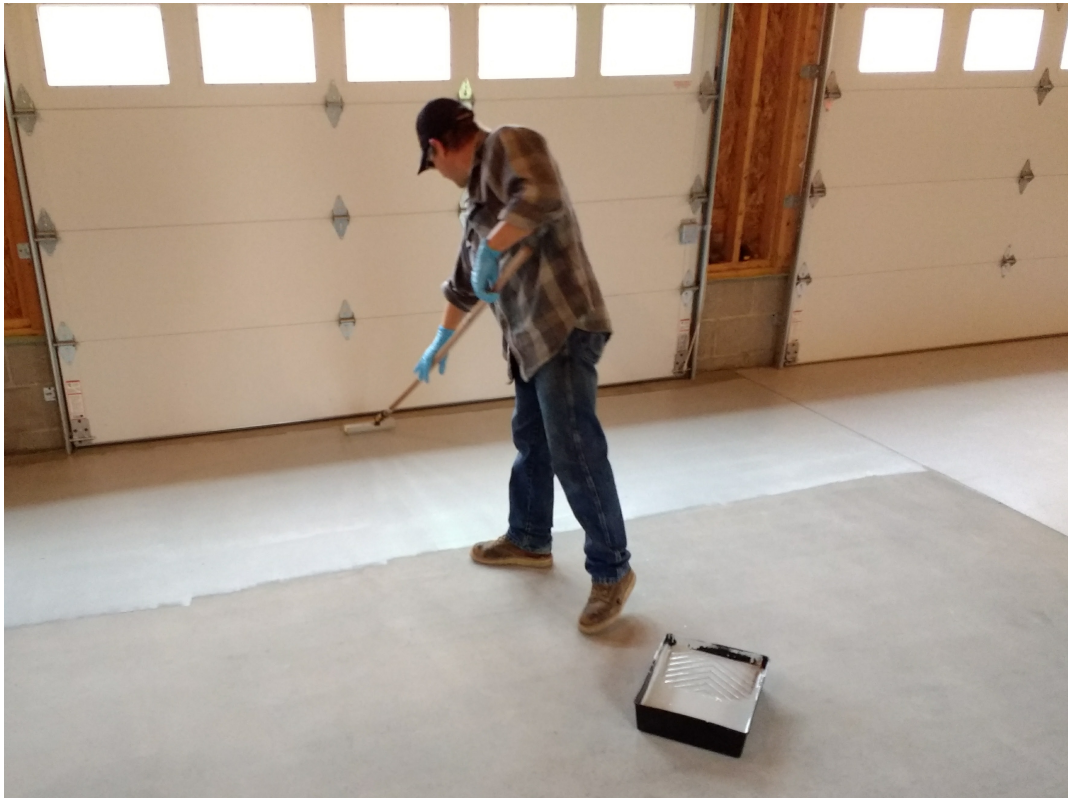
Figure 1. Application Of Biobased Industrial Floor Coating By Roller
