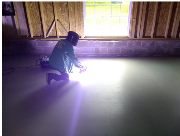
Figure 3. Quick Cure Of Biobased Coating Spot Repair Using Handheld UV Cure Lamp
